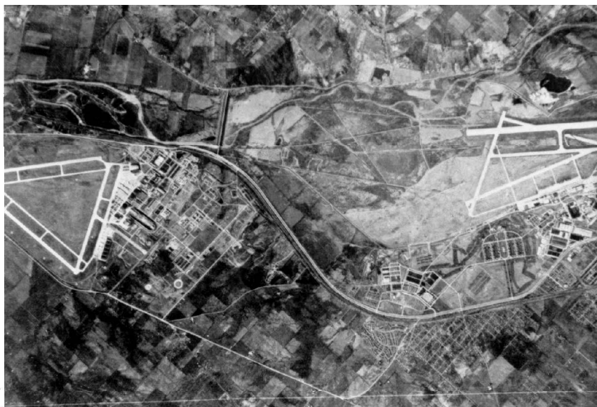
Fig. 4. Wright-Patterson AFB, the complex of organizations located at Dayton, Ohio. Wright Field, the top secret engineering research facility is located at the triangular field on the left. Patterson Field, the actual air force base is separated by a civilian highway and is on the right. Howard McCoy's Intelligence Division was located right of center in the picture on Patterson Field. (USAF)
